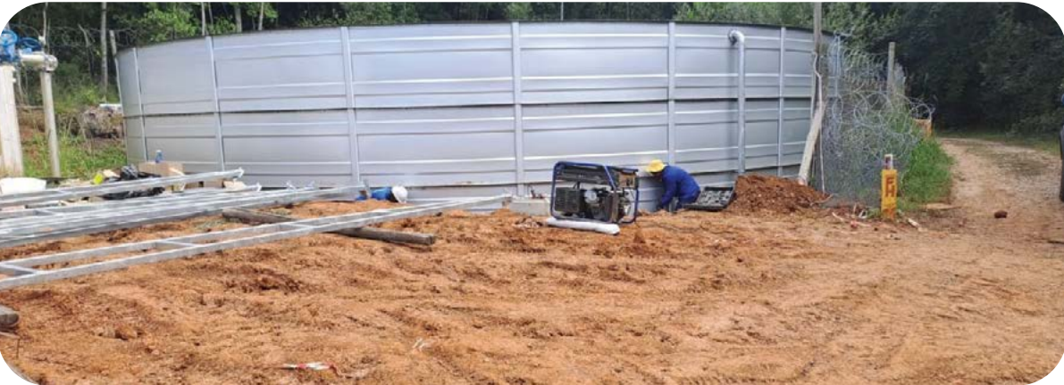
Figure 42: New infrastructure to promote sustainable water use
